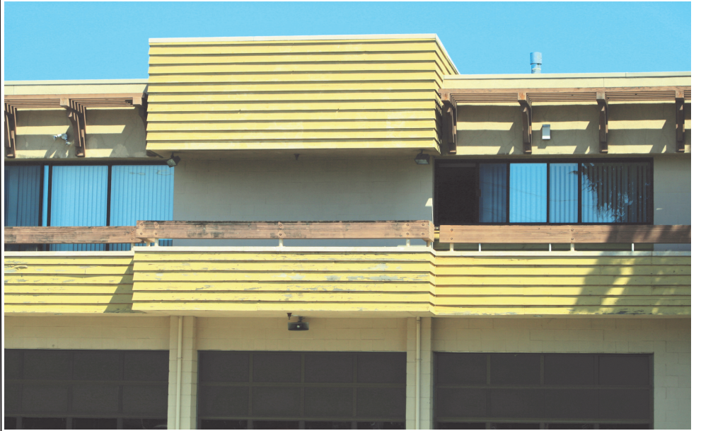
The Essence of Cotati: Rancho Adobe Fire Station. This fiscal year, the Cotati Redevelopment Agency will spend $4.3 million. Between 2010–2014, they plan to spend over $18 million. For years, the Fire District has asked the city for $50,000 of these funds to replace the warped siding on this blighted building, which is literally at the heart of town. The city constantly refuses, but loves to spend your property tax money on traffic calming, urban infill, and other new-agey clichés.
